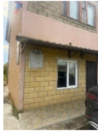
Shirak Administrative Office
