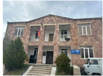
Jrarat Administrative Office
