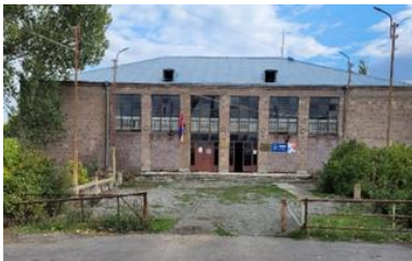
Gharibdjian administrative office
