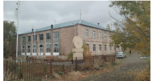
Kaps Administrative Office
