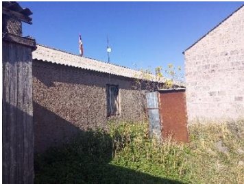
Kamut Administrative Office
