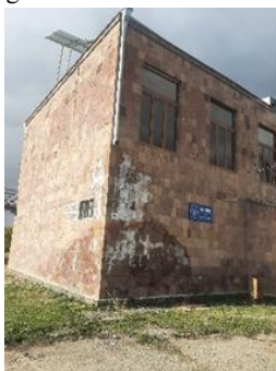
Yerasgavors Administrative Office
