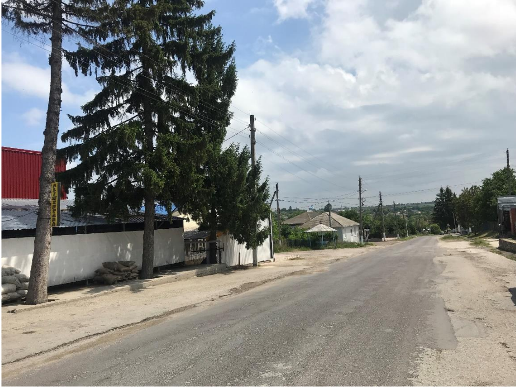
Photo 7. The lighting of the main street
