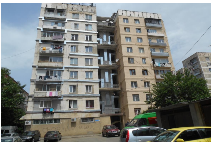
Picture 5. The pilot residential building in Temka district
