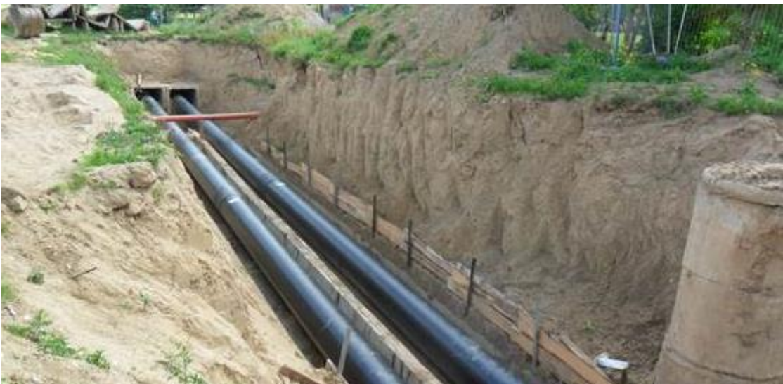
Image 10. Trenchless installation of heat supply pipe networks
