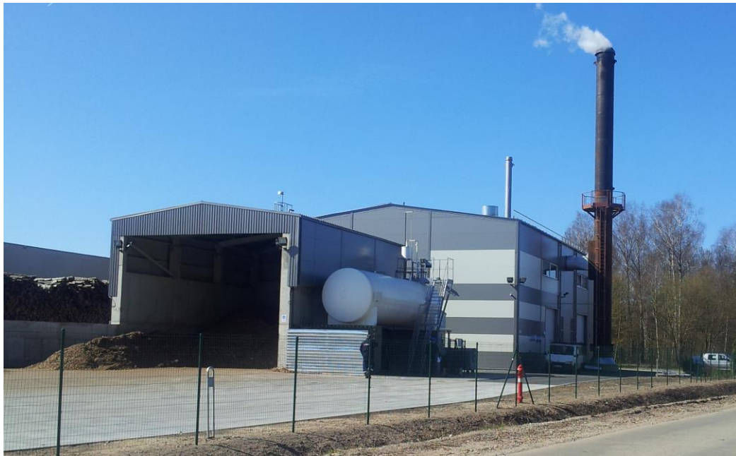
Image 8. Biofuel-powered boiler house
