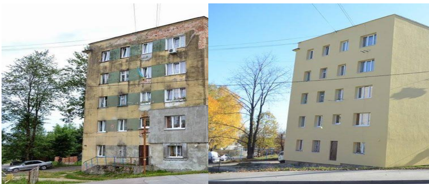
Image 11. Tower block before and after renovation
