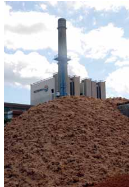
A biomass storage in the Żerań Heat and Power Plant. Phot. from the archives of Vattenfall
