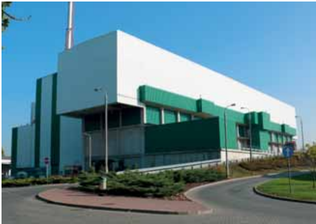
Municipal Solid Waste Incineration Plant Phot. from the archives of the Municipal Solid Waste Incineration Plant.
