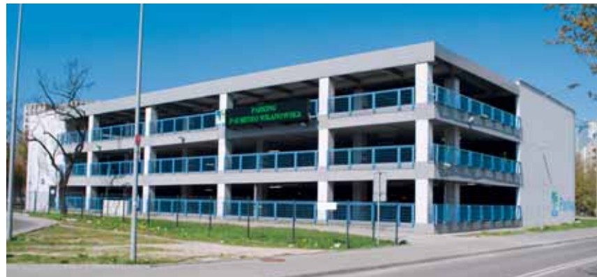
P&R car park. Phot. S. Sadowski (the Roads and Public Transportation Department)
