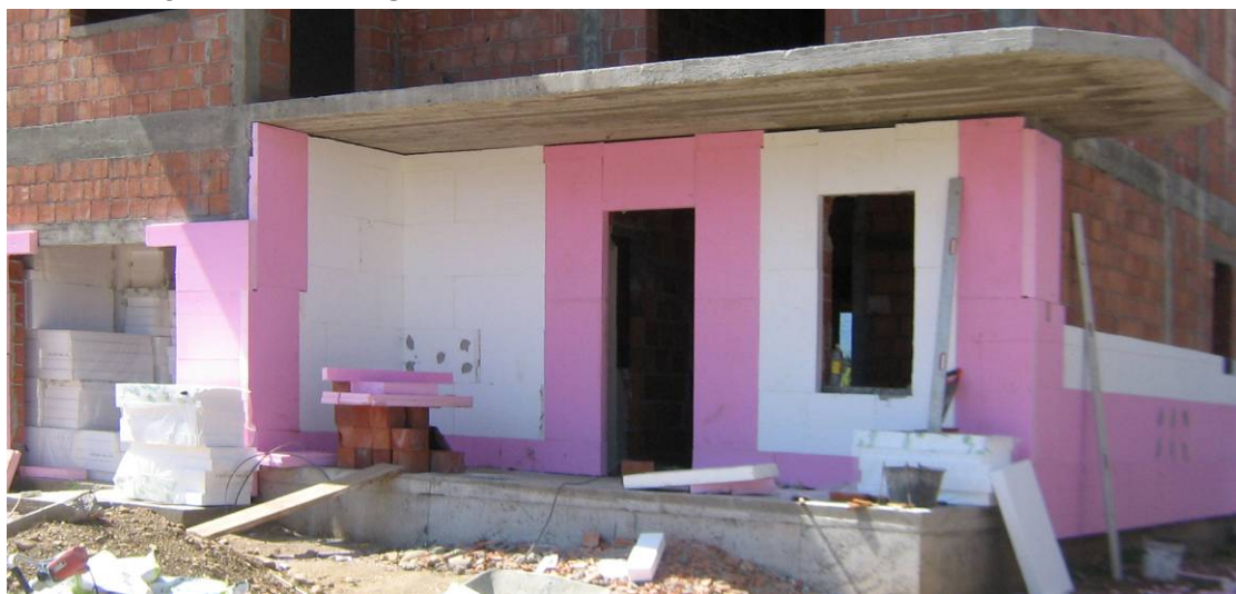
Figure 2.3: Thick External Insulation Layer in New Building in Breza
