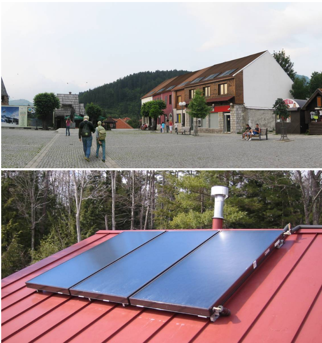
Figure 2.4: Examples of Installation of Renewable Energy Plants
