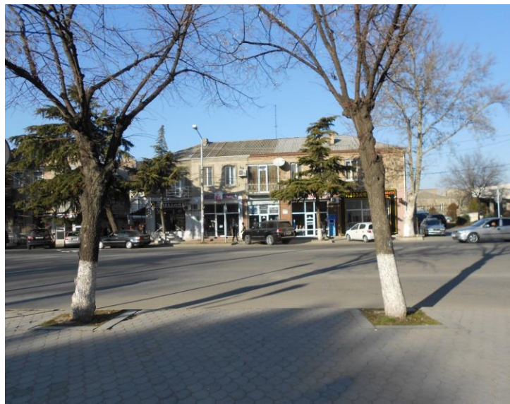
Picture 12. Two-storey residential building (39 I. Chavchavadze str.)
