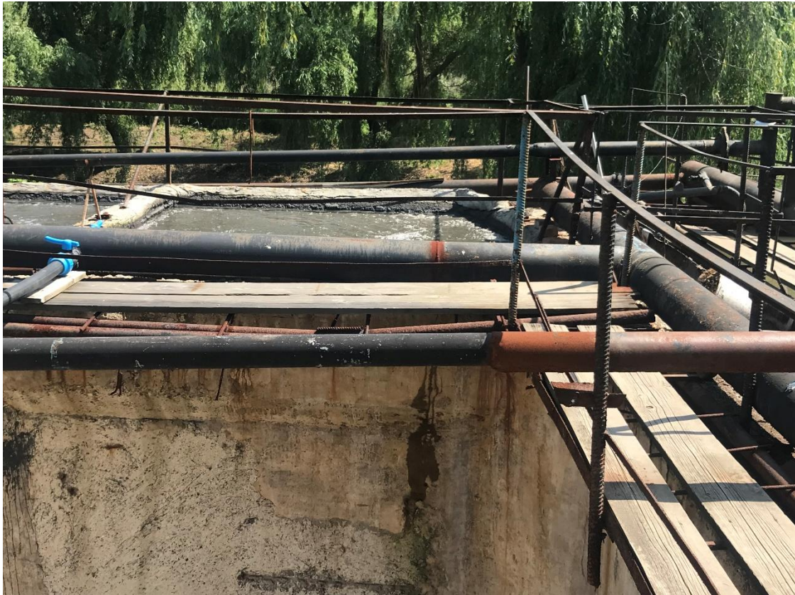
Photo 7. Current state of the wastewater treatment plant
