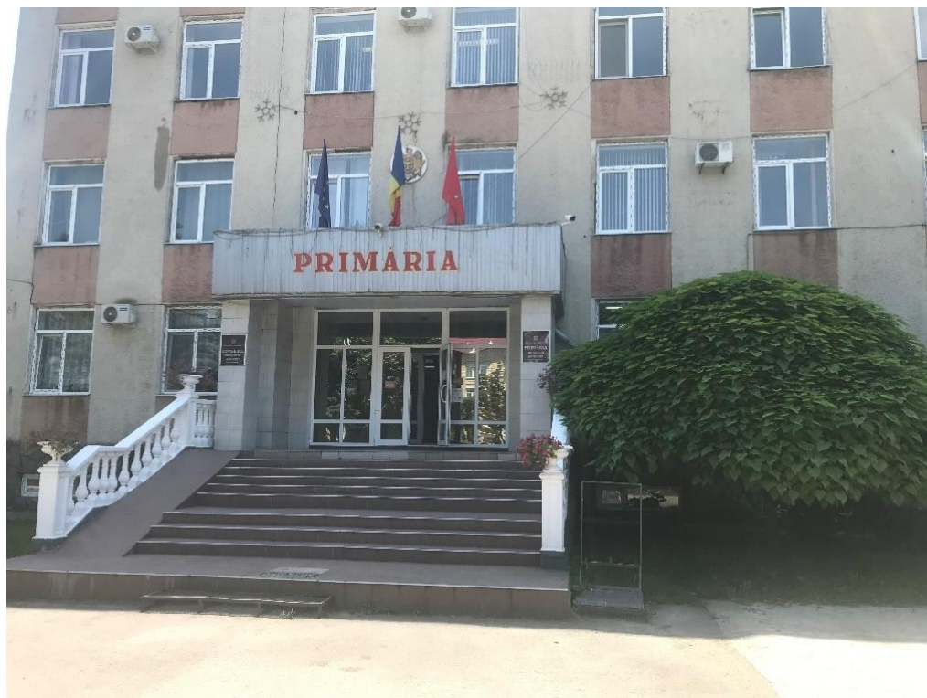
Photo 1. City Hall Building
