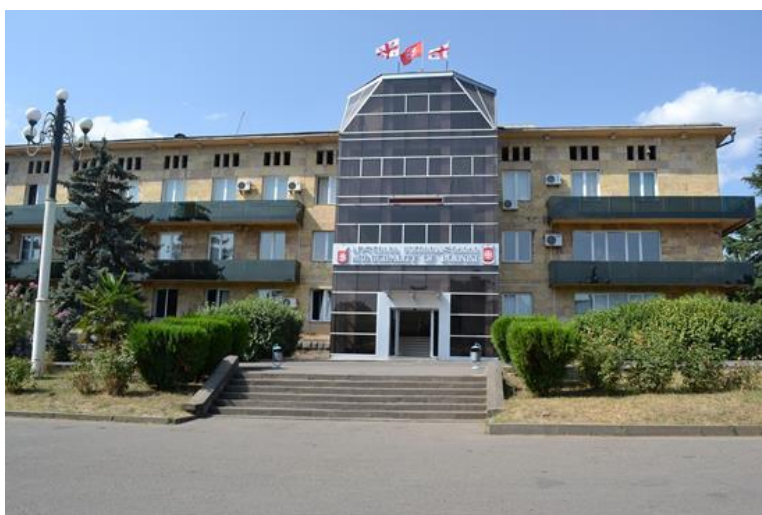
Picture 2. Building of Bolnisi Municipality City Assembly
