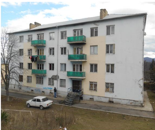
Four-storey residential building (Address: David Agmashenebeli str.N 41)
