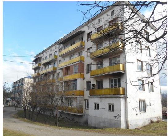
Five-storey residential building (Address: David Agmashenebeli str.N 39)
