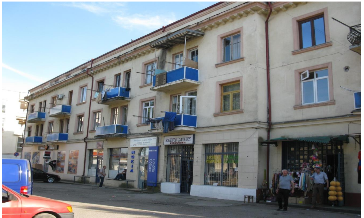
Picture 11. Three-storey Residential Building (6 Tabukashvili St.)
