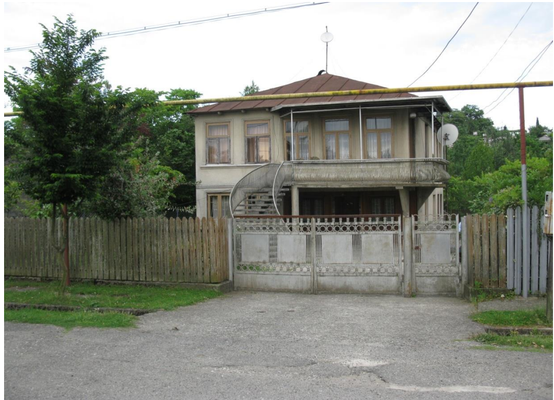
Picture 7. Private Residential House (13 Antelava St.)
