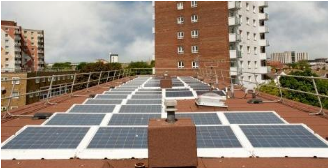
Solar Panel Installation at Whatleigh Gardens, Poole
