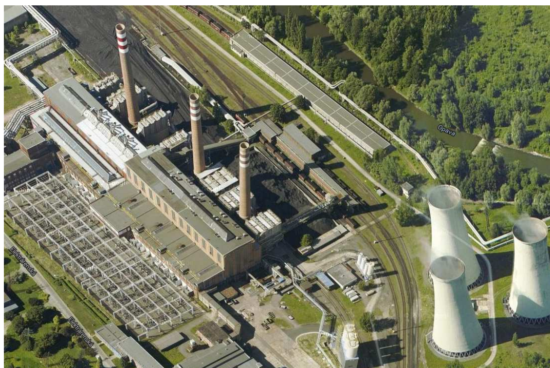
Figure 20: Source of Dalkia Česká republika - Třebovice Power Plant – air view (Google maps)
