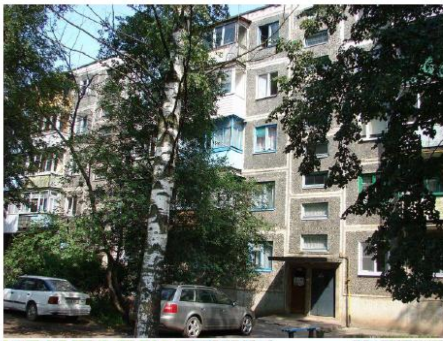
Figure 3. Block of flats No. 23 in Marinenko street.
