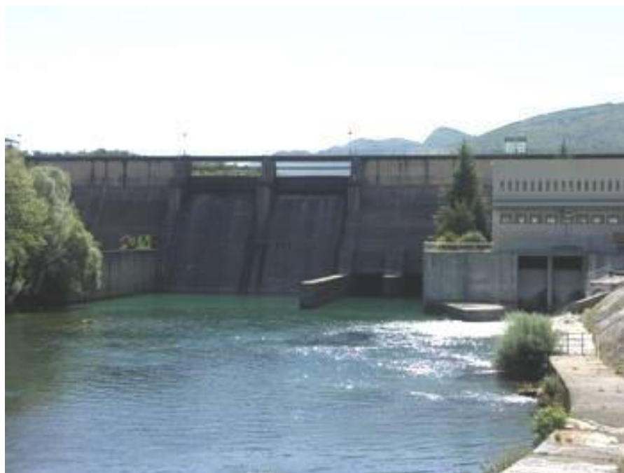
Figure 12.2: Hydro power plant, HPP Trebinje 2
