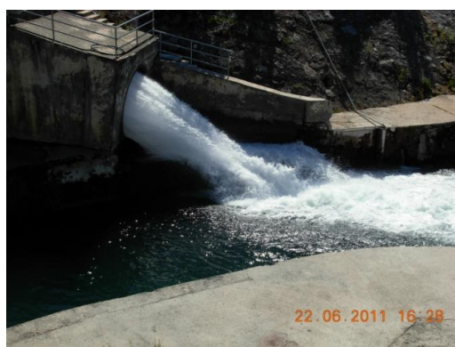
Figure 10.1: Outlet for biological minimum on the HPP Trebinje 2 for the river Trebišnjica
