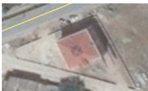
FIGURE 5: TOP ROOF OF MUNICIPALITY BUILDING
