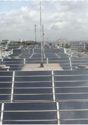
Solar panels on the OPAC building Rue de Plantes, 14 th district.
