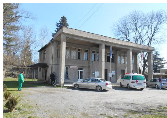
Administration building of village Naphareuli
