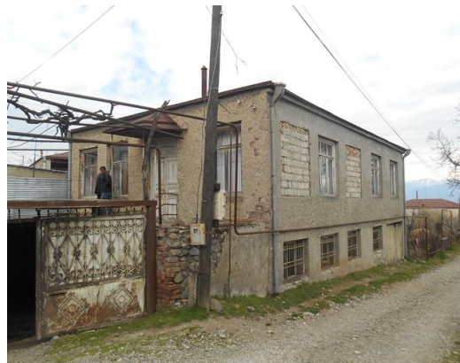
Private residential house in village Busheti
