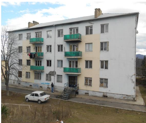
Four-storey residential building (Address: David Agmashenebeli str.N 41)
