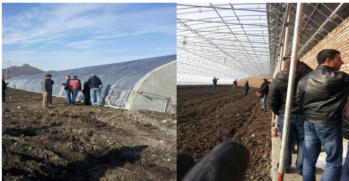
Picture 6. A Solar Energy Consuming Energy-efficient (Chinese) Greenhouse in Marneuli
