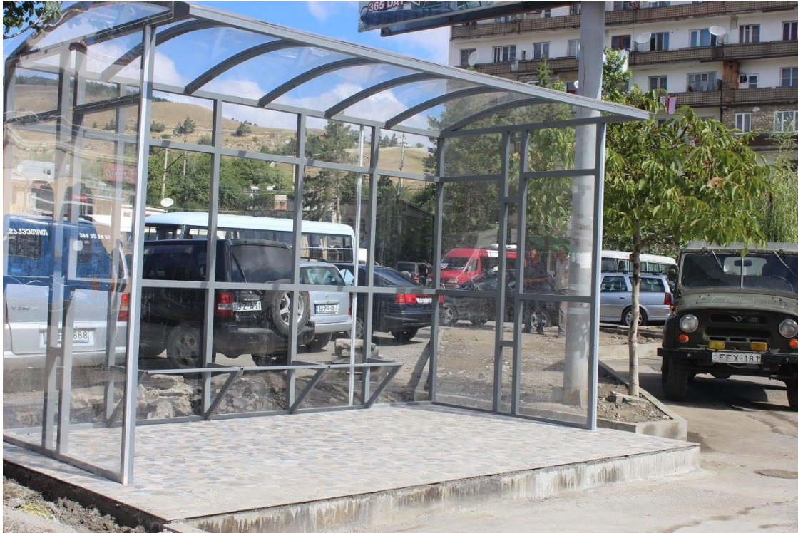
Picture 4. Passenger transport stop-station at the Akhaltsikhe bus station neighboring territory
