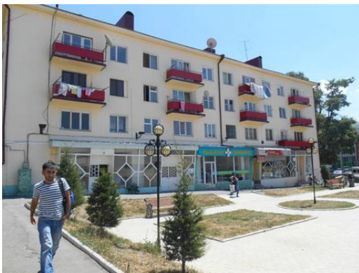
Four-storey residential building (1, Shalva Akhalsikheli st.)
