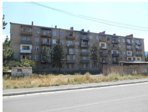
Five-storey residential building (42, Aspindza st.)
