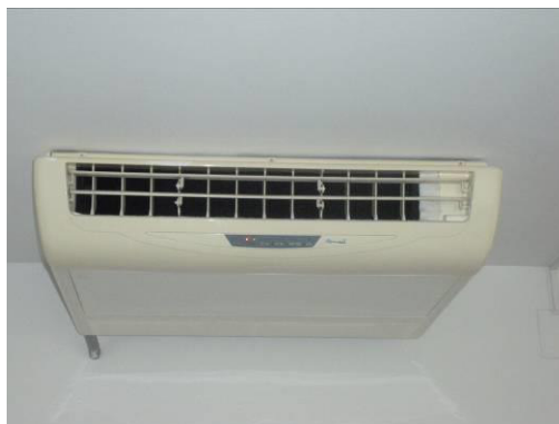
Figura 4. Unitat terminal split
