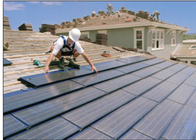
FIGURE 9: PHOTOVOLTAIC SOLAR ENERGY
