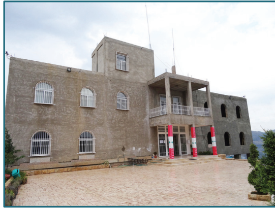
FIGURE 5: BAAKLINE MUNICIPALITY BUILDING
