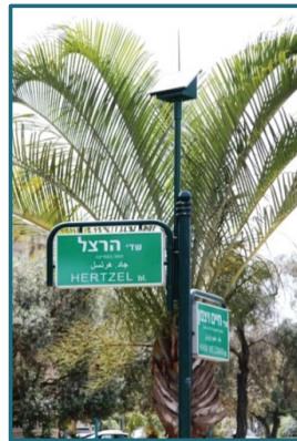
Figure 8 –Solar lighting post in Ramla
