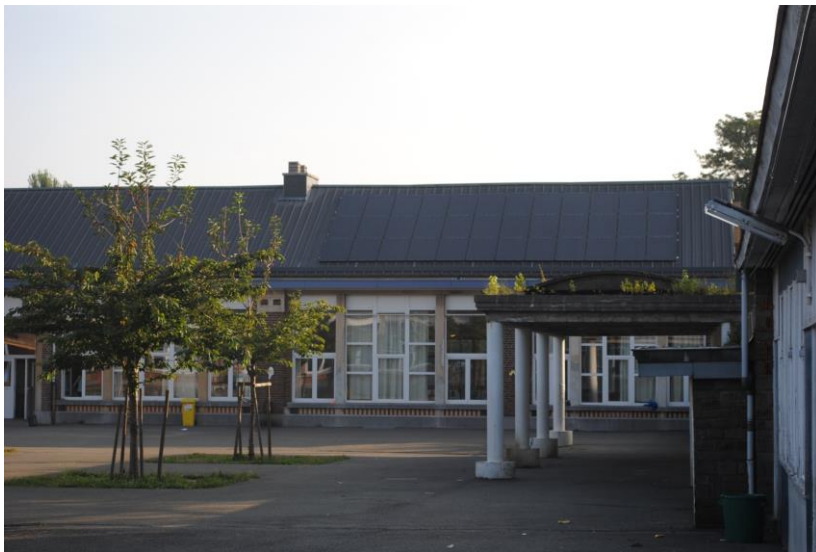
Photovoltaic installation 2 at Distexhe school
