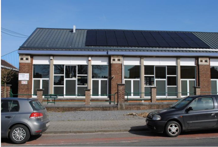
Photovoltaic installation 1 at Distexhe school
