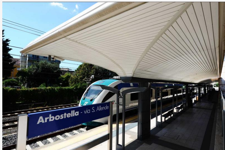
The Metro station "Arbostella"
